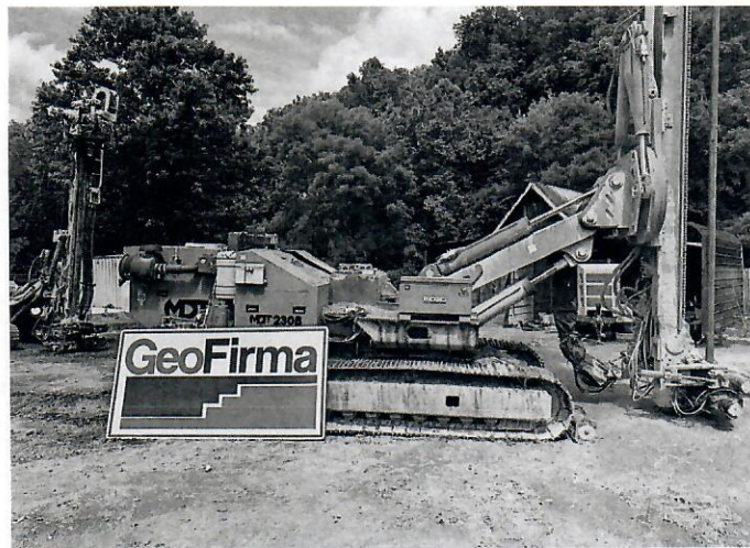
Fig. 1. Ground anchors are installed with a specialized drill. (Photo courtesy of GeoFirma, LLC)
