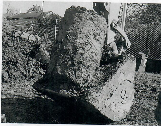
Extraction of Top of Column
