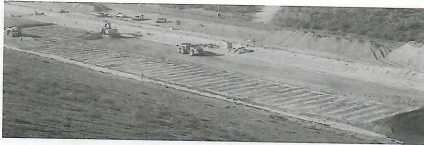
Top of CDSM cells exposed for placement of filter and drain
