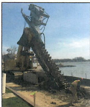
Photograph 2. “One Pass” Trenching equipment (Courtesy of DeWind)
