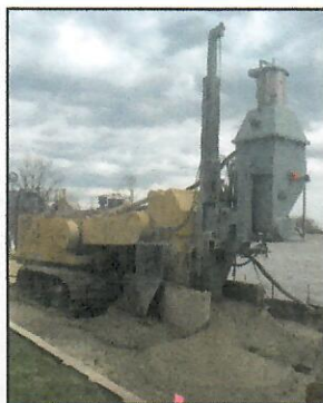
Photograph 2. “One Pass” Trenching equipment (Courtesy of DeWind)
