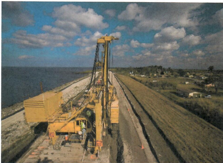
Photograph 1. TRD in use at Herbert Hoover Dike, FL (Courtesy of the Keller Group)
