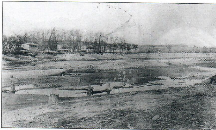
Figure 2. Photo showing East Reservoir drained after 1913 dam failure (Photo courtesy of Cuyahoga Falls Library)
