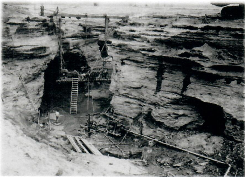
Photo 4. Major karstic features in the foundation, Wolf Creek Dam, KY. (Courtesy of USACE.)
