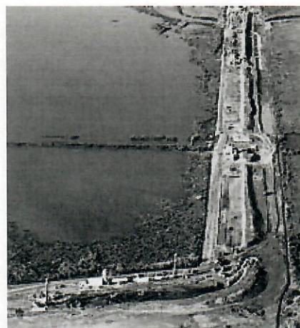
Photo 6: View of LPVIII Deep Mixing.
