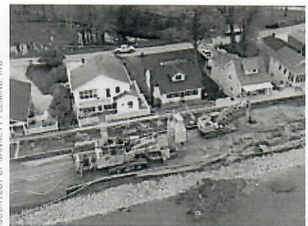
Photo 9: Installation of the DM cutoff using the "One Pass" system.
