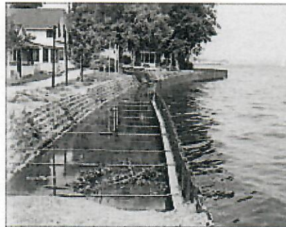
Photo 8: The shoreline of Buckeye Lake Dam, Ohio before remediation.
