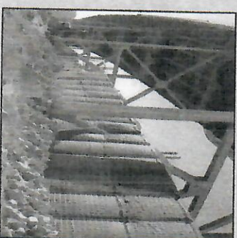
Temporary Sand Baskets at Valtia Bar Dam
