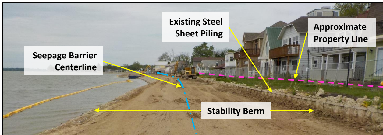
Figure 4: Stability Berm Construction
