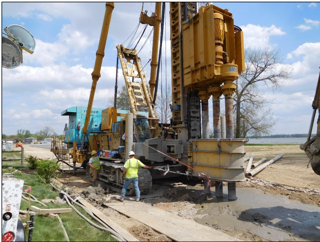
Figure 5: Raito Wet Rotary Shaft Mixing Equipment
