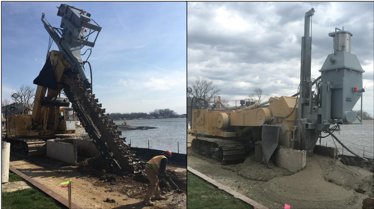
Figure 6: Dewind Onepass Rig – Bar/Chain Entry on Left, Mixing Position on Right
