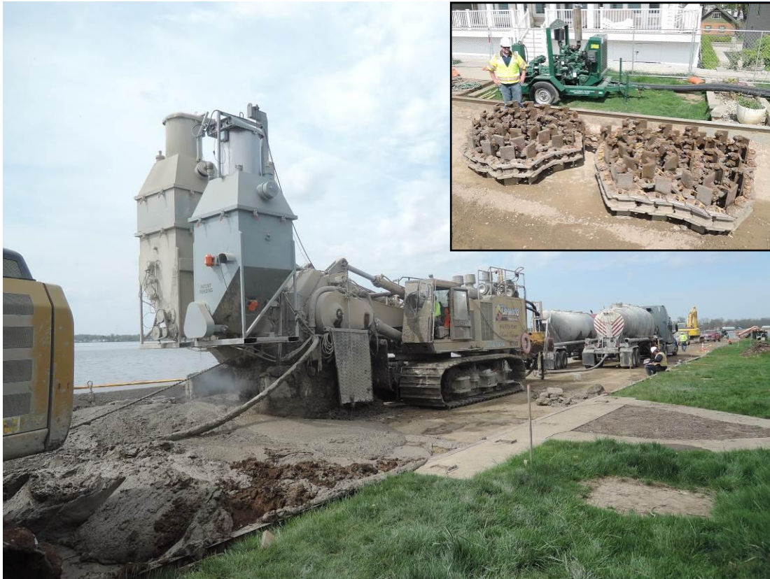
Figure 4. Chain-saw type mixing equipment in operation, with post and chain in the ground, binder hoppers above the post and chain, wet-mixed spoils behind the mixing rig, and inset showing toothed chain.
