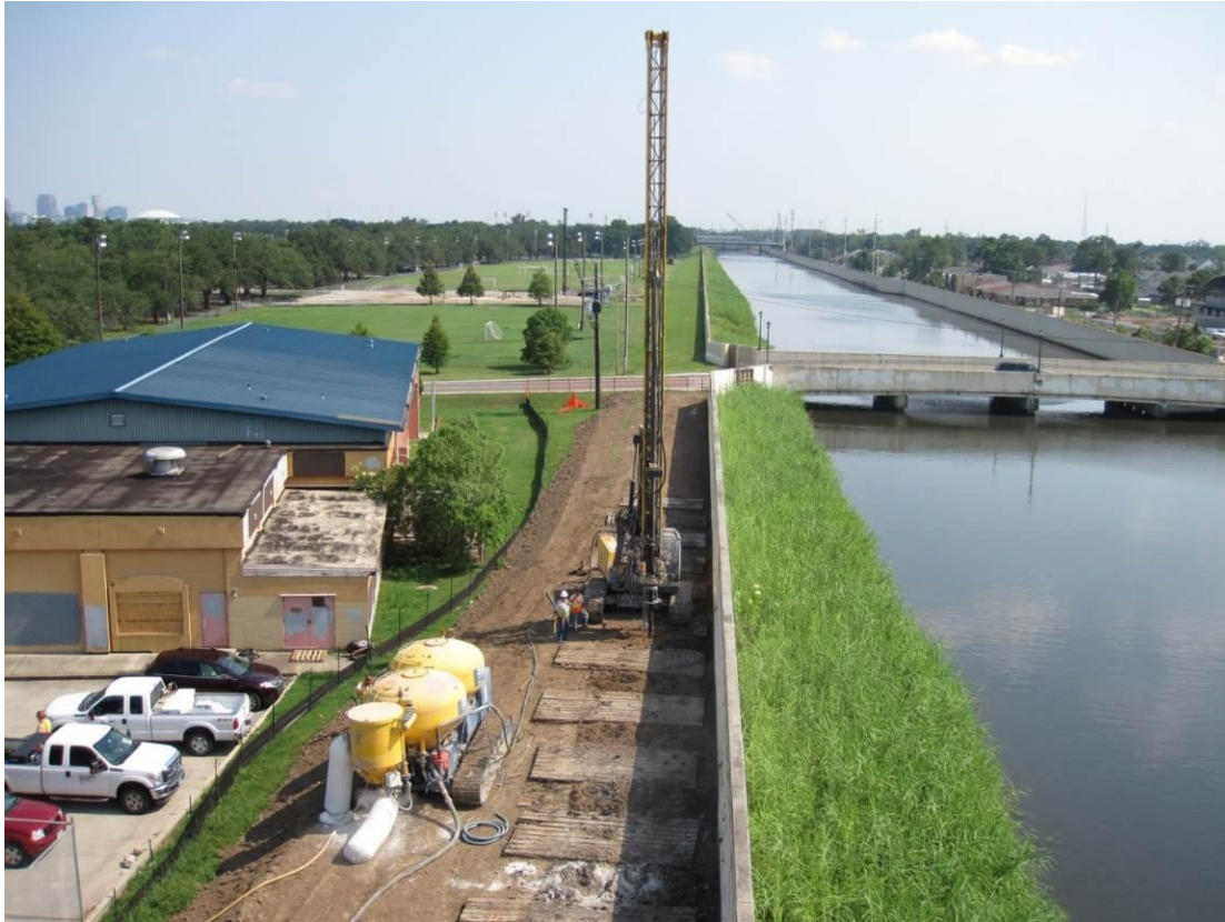
Figure 2. Deep mixing by the dry method using single-shaft, vertical-axis equipment at Orleans Avenue Floodwall in New Orleans. (Photo courtesy of Hayward Baker Inc.)
