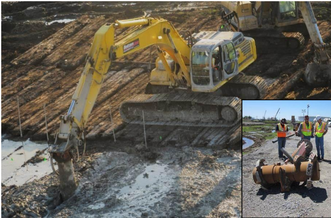
Figure 5. Horizontal axis rotary drum mixing underway using the wet method, and inset showing mixing drum. (Main photo courtesy of Hayward Baker Inc.)
