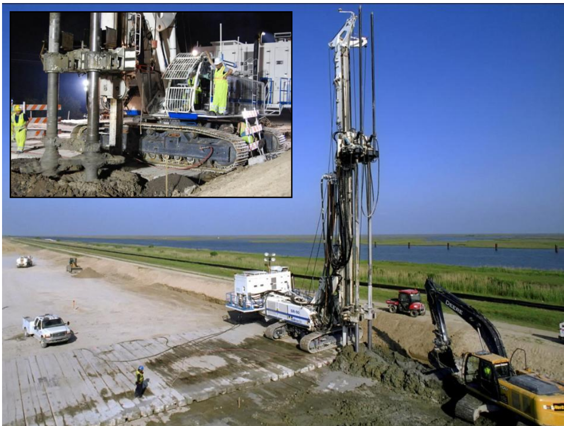
Figure 1. Deep mixing by the wet method using twin-shaft, vertical-axis equipment at earthen levee LPV 111 in New Orleans. Inset shows mixing blades in operation. (Photos courtesy of TREVIICOS).
