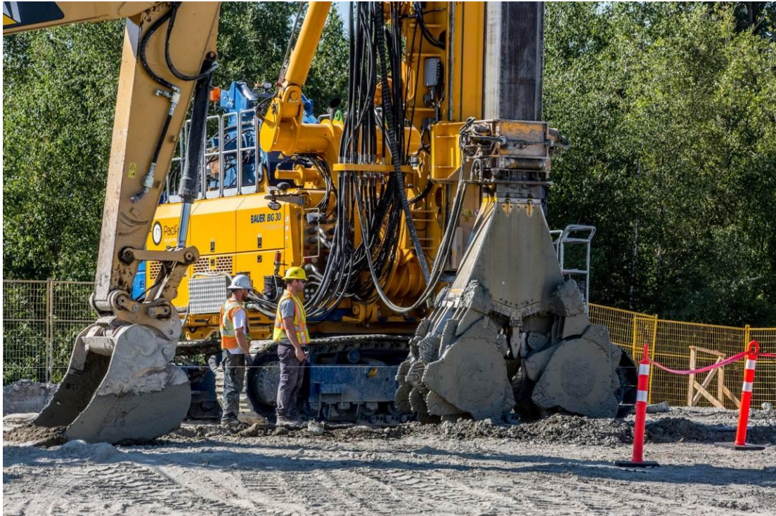
Figure 3. Cutter soil mixing equipment. (Photo courtesy of Pacific Ground Engineering)
