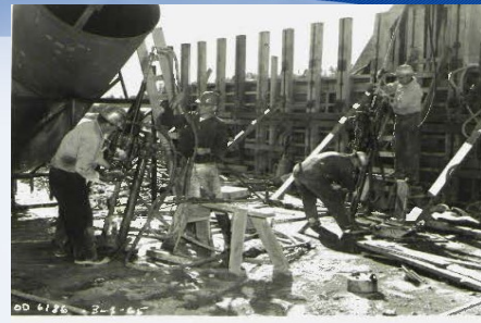
Photo No. 30. Drilling curtain holes through concrete at Elevation 128 in monolith 19. View downstream. Neg. No. 0D 6186 2-4-65 (Courtesy of California Department of Water Resources)
