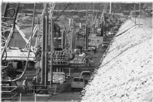
Protective Concrete Embankment Wall Wolf Creek Dam, KY
