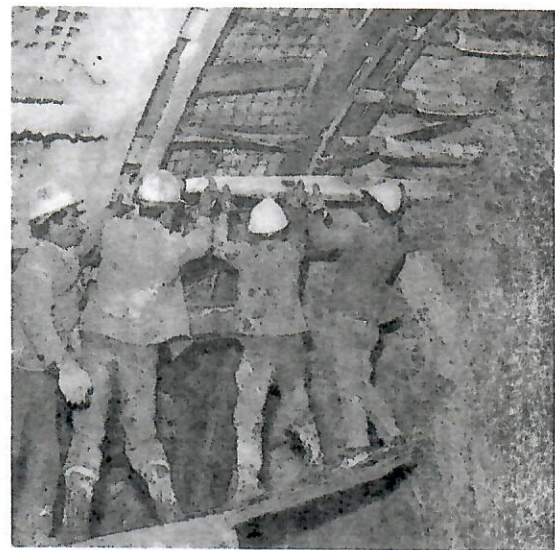
Photograph 4 - Infilaggi being placed in predrilled holes, Limina Motorway Tunnel, Mammola, Italy.
